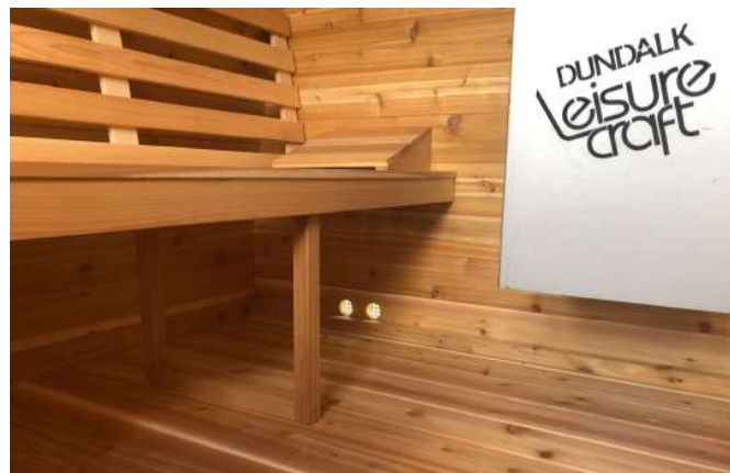
Inlet beside wood heater on Back wall
