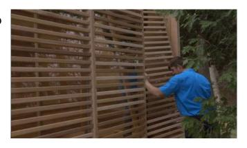
Once the front panels are assembled together, secure the last panel to the corner post in the same method as previous steps.
