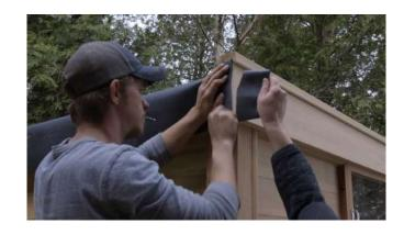
Tuck the membrane under the lip of the roof and secure with a finishing nail.
