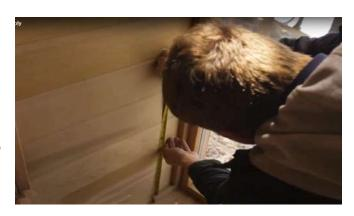
Install the supplied support screws into your marks as shown. Screw them in until they are about ¼" (6mm) out of the wall.
