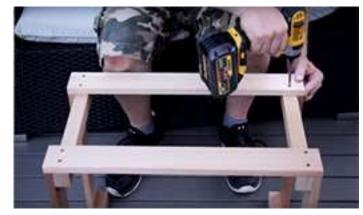
Place assembled heater guard around electric heater and screw to wall using (4) 2 ½" (64mm) screws.
