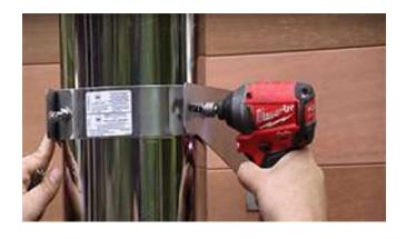
Attach the chimney cover plates starting with the bottom plate, using 1 ½" (38mm) screws ensuring the top plate overlaps the bottom and that they are level
