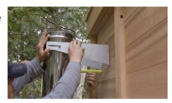
Tighten up the chimney support brackets with a 7/16" (11mm) socket or wrench until snug.
