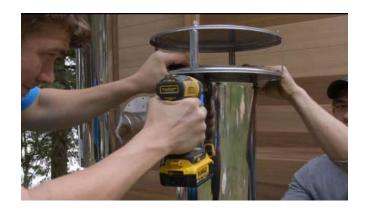
Attach chimney top onto the chimney and secure them together with the provided screws.
