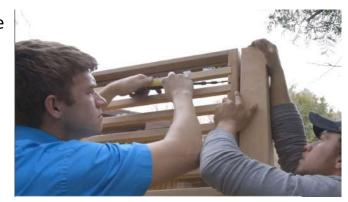
Install the door plugs by pushing them into the pre drilled holes then tapping them in tight with a rubber mallet.
