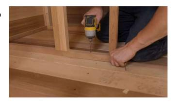
Secure the bench supports to the top bench from underneath using 2 ½" (64mm) screws.
