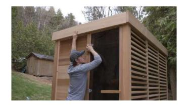
Place your EPDM membrane on top of the sauna. Spread it out evenly over the entire roof.
