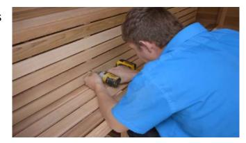
Before putting on the lower bench enclosure, slide the backrest supports behind the top bench.
