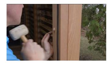
Attach the wider trim pieces over the seams of the sauna using the provided finishing nails.
