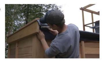
Place the back trim piece up tight under the edge of the roof.
