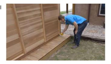
Once the sauna walls are overhanging 1 ½" (38mm) on all sides of the floor, use 2 ½" (64mm) screws to secure to the base through the pre drilled holes.
