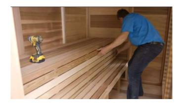
Secure the Front bench enclosure to the bench supports between the slats using 2 ½" (64mm) screws.
