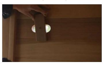
Install the cedar vent cover over the outlet holes on the inside of the sauna with a 1 ½" screw.
