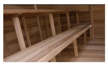
Secure the bench supports to the bottom bench from underneath using 2 ½" (64mm) screws.
