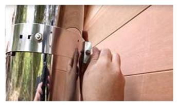
Attach chimney support braces to the support strap and thread the nuts on hand tight.
