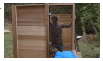
Secure the side wall panel to the glass door using the 2 ¾" (70mm) Connector lag screws through the predrilled holes.
