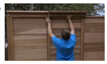
Inside, line up the holes and fasten the roof panels together with 2 ¾" (70mm) connector bolts and connector cap nuts.
