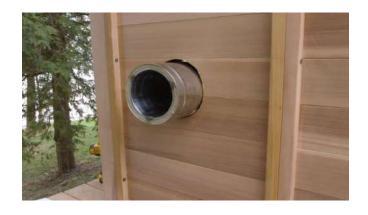
Insert the "T" connector to the short connector ensuring it is straight.
