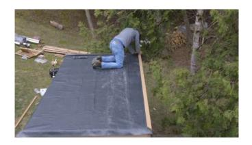
Line up the roof cap pieces so the corners are tight together and tap them down tightly over the trim pieces with a rubber mallet.
