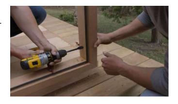
Secure the door frame to the last corner post using the 2 ¾" (70mm) Connector lag screws through the pre drilled holes.
