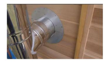
Attach the rain guard to top chimney piece and secure with provided screws.
