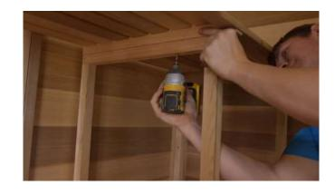
Position the bottom bench on top of the lower section of the bench supports.
