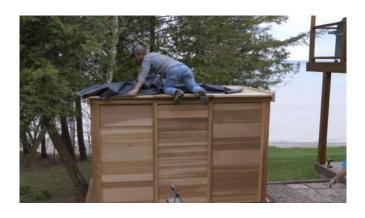
Once the membrane is laid out evenly over the top of the sauna, use staples or nails to secure it to the trim pieces.
