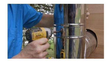
Wrap the chimney support strap around chimney and use the provided nut and bolt to secure.
