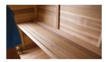
Line up the remaining bench supports with the braces on the bottom of the top bench.
