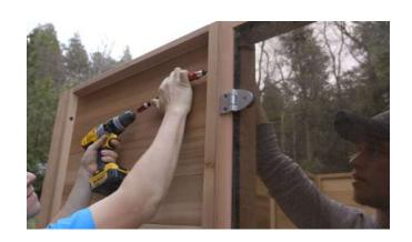
Before attaching the corner post to the door, pre drill pilot holes in the frame of the door to prevent splitting.
