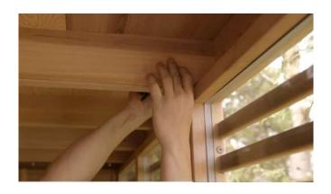
When you have the roof panels connected, tighten up the bolts with a drill and hex key.
