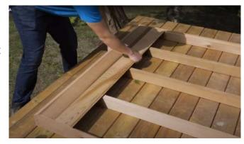
Fasten the floor boards into the floor joists and the inner floor joists with 1  $\frac{1}{2}$ " (38mm) screws.
