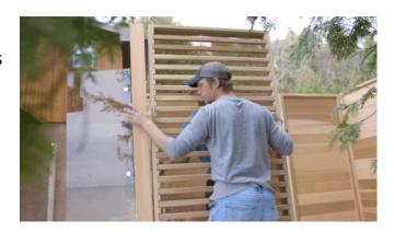
Make sure the next window panel is flush to the first one and fasten it together with 2 ¾" (70mm) connector bolts and a connector cap nut.
