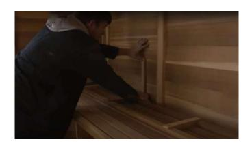
Ensure they align flush behind the bench supports and secure with 2 ½" (64mm) screws.
