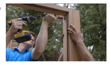
Line up one of the window panels flush to the corner post and secure it using the 2 3/4" Connector lag screws through the pre drilled holes.
