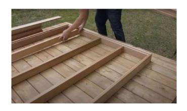
Once the floor joists are spaced out evenly, secure them through the pre drilled pocket holes using 2  $\frac{1}{2}$ " (64mm)screws.
