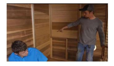
Ensure the bench supports are tight to the side and back walls, then secure the supports to the walls and floor using 2 ½" (64mm) screws.
