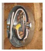
Recommend low profile "pancake box" rather than standard octagon box. This can be surface mounted flush inside of the sauna with light fixture fitting over the box.
