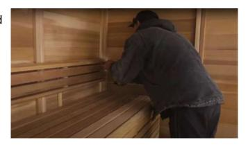
You can now secure the lower front bench enclosure to the bench supports by screwing between the slats using  $2 \frac{1}{2}$ " (64mm) screws.
