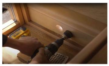
If an electric heater is chosen, Drill inlet holes centered under the heater close to the floor.
