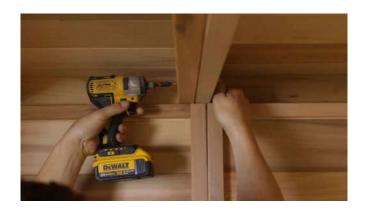
Line up the roof panels to the edge of the walls and secure using 2 ½" (64mm) wood screws.
