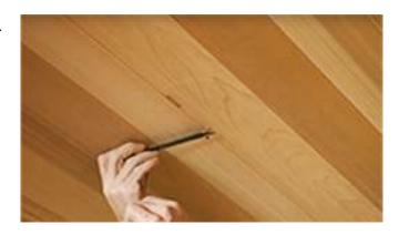
Start a hole inside your circle with a drill bit or other method, then use a reciprocating saw or jig saw to cut out the circle as neat as possible.
