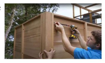
Secure the side wall to the post in the same manner ensuring that the outside of the wall is flush to the post.
