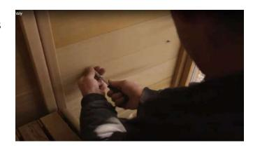
Hang the electric heater on the screws.
