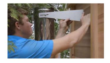
With the nuts on the side of the straps loose, level up the chimney pipe.
