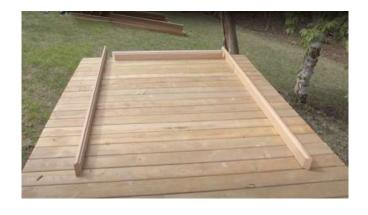
Secure the corners of the floor supports together using 2 ½" (64mm) screws in the pre drilled holes.
