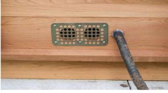
Install 1 of the stainless steel vent grills over the inlet holes on the outside of the sauna centered over the holes using  $1 \frac{1}{2}$ " screws. (38mm) (6pcs)
