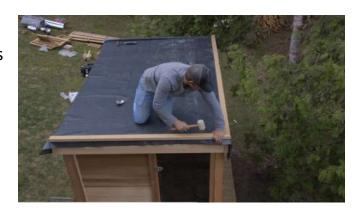
Using the supplied finishing nails, secure the roof caps into place.
