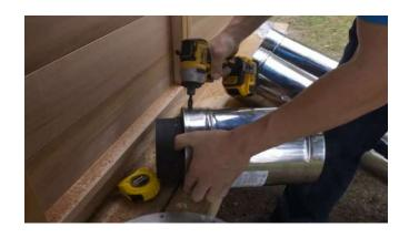
Slide the assemble pipe through the hole and into the stove.
