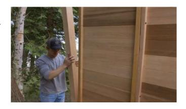
Position the walls onto the base ensuring there is 1 %" (38mm) overhang on each side.
