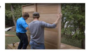
Connect the wall panels together using 2 ¾" (70mm) connector bolts and a connector cap nut.
