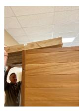
Connect the heater wires, then lay the wire into the groove that is cut into the roof section. This will ensure that the dust cover can be reinstalled without interfering with the wires (21). Be sure that the wires plugs are fully connected and seated securely into the receptacles (22). The plug accompanying your Hampton sauna will be different than pictured (23). Feed the power connector through the hole in the dust cover and reposition the dust cover over the roof section (24).
