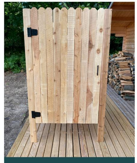
12. The shower is designed to be free standing, but if you desire added rigidity, you can screw legs or wall(s) to the floor or adjoining structure as desired.
