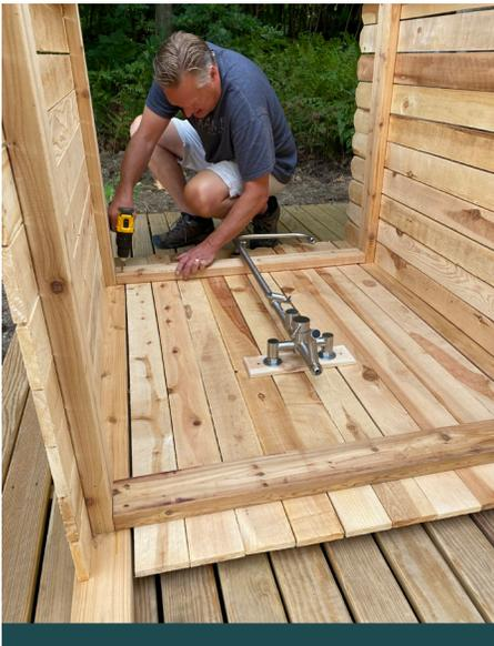
4. Push the horizontal supports on the side walls tightly against the horizontal supports on the rear wall and screw into place using the 3" screws. (Holes are pre-drilled and screw will enter at a slight angle.)
