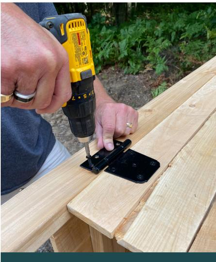
10. Allow for approximately a 1/8" gap between door and side wall and screw the door into place with provided screws. Note that there will be a larger gap of 1/4" +/- on the opposite sidewall.
