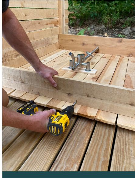
8. Screw the shelf in place with 2" screws through pre-drilled holes. The shelves will bring stability to the structure.
