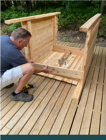
7. Position the lower shelf in place with rough-side facing up. It, too, can be mounted either below the horizontal supports or above, whatever your preference. Again, be sure the side walls are tight to the shelf before installing screws.
