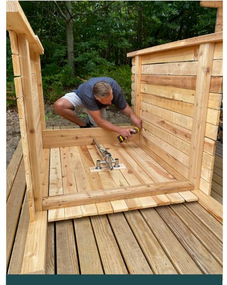
6. Screw the shelf in place with 2" screws through pre-drilled holes. Be sure the side walls are tight to the shelf before installing screws. The shelves give stability to the shower.
