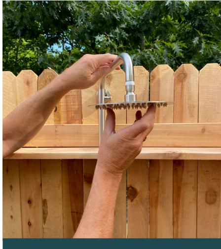
14. Turn shower head onto fixture and gently tighten with wrench.
