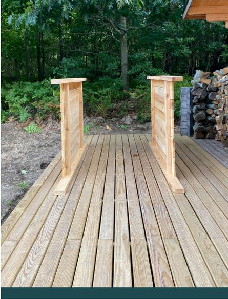
1. Set up the two side walls on edge as shown. Be sure the ends with the door stops are facing up.
