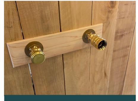
18. The other outlet comes capped from the factory. (If you wish to have your plumber run hot and cold water to the shower, then he will remove the cap, swivel, and adaptor fittings so that he can connect to the 1/2" water lines.)
