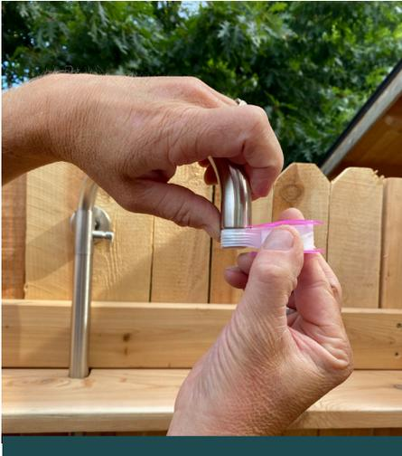
13. Wrap threads of shower head with sealing tape. (Always wrap clockwise)
