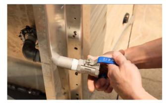
Remove the valve from the plastic packaging and thread it onto the end of the long pipe.
