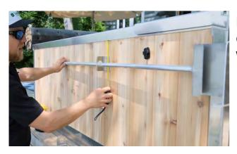
Place the ash scoop brackets (if ordered) in the desired location ensuring they are level and secure with 2 – 1" (25mm) screws per bracket.
