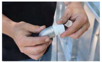
Screw the short pipe into the elbow.
