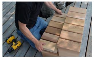
Flip the assembled stairs right side up and then repeat the process to attach the bottom step.
