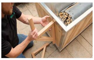
To install the roll up cover, secure the cover brackets onto the end of the tub opposite the heater and secure with  $2 - 2 \frac{1}{2}$ " (64mm) screws into each bracket.
