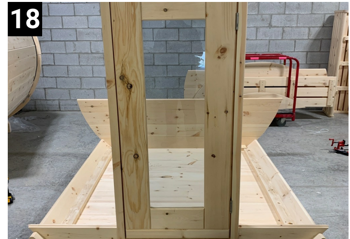
18 Insert door with hinges to right
