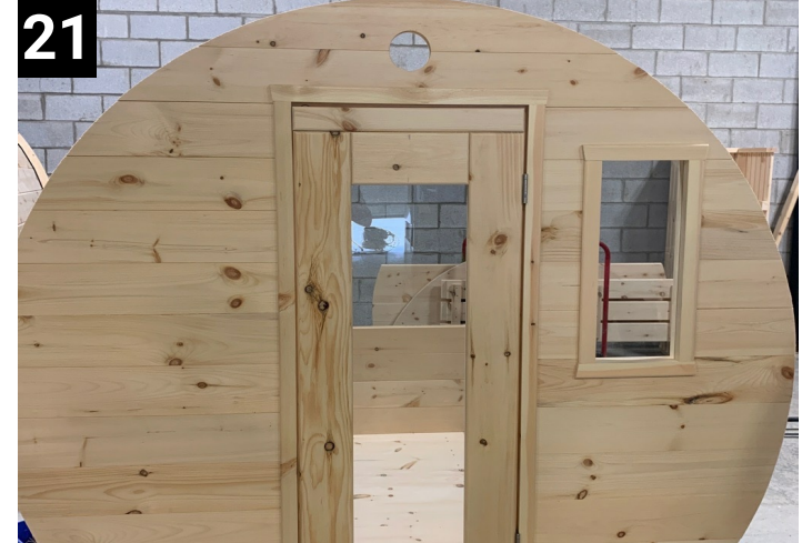
21 Put top pc of wall over door and fasten with 4" screws
