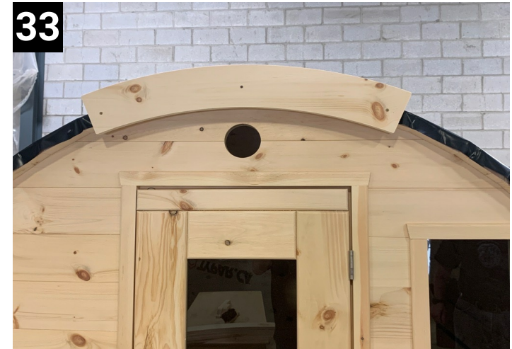
33 Attach barge boards. Center top one and fasten on.
