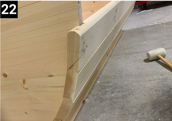
22 Put a total of 4 staves on each side now and fasten into wall
