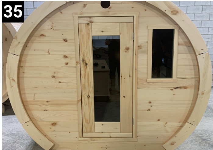
35 Do same process for back barge boards
