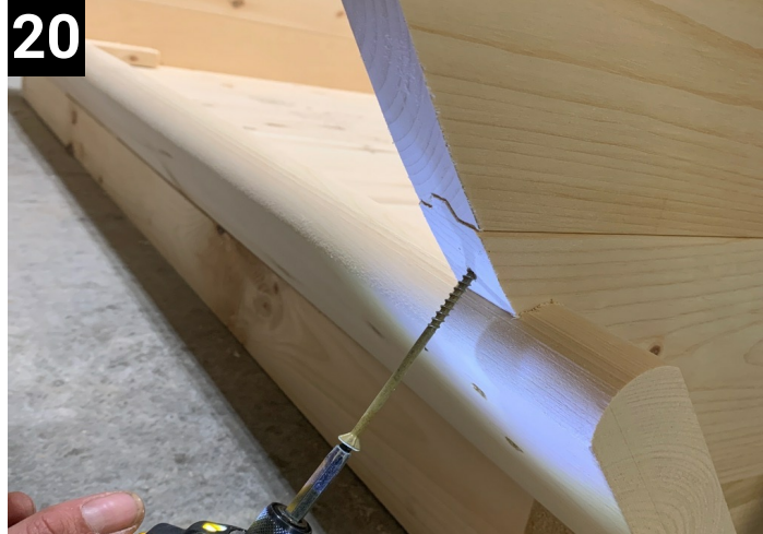
20 Screw wall together with a 4" screw
