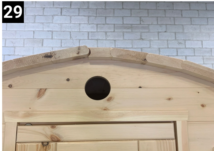
Set top stave in and then close up staves tight. Screw all staves down with screws now
