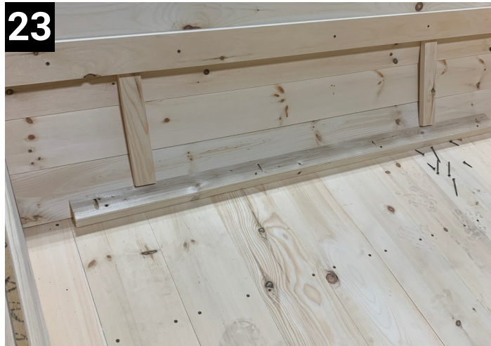
23 Using bench height measuring sticks fasten Ben h support cleat
