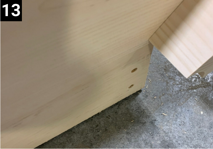
13 Front wall and back wall should over hang floor at both ends
