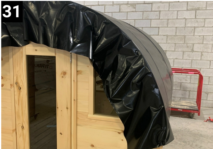
31 Put roof membrane over and make it even down both side. Staple over front staves
