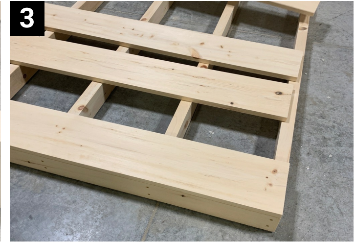
3 Lay floor boards on and start at one end and screw it down. Keep floor boards as tight together as possible
