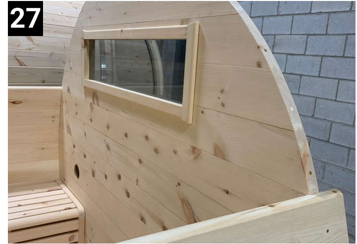
Add rest of back wall and fasten with 4" screws
