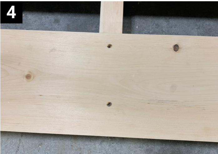
4 2 screws into each floor base. Leave Center long board with no screws. Walk isle area.
