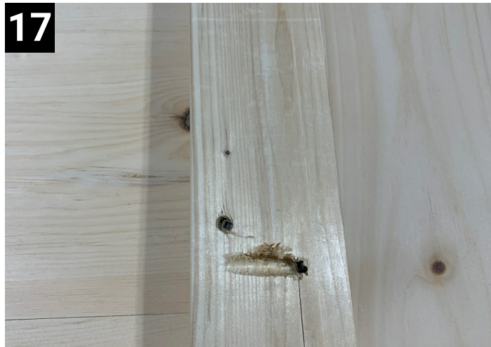
17 Make sure to put screw to inside so not to miss floor frame
