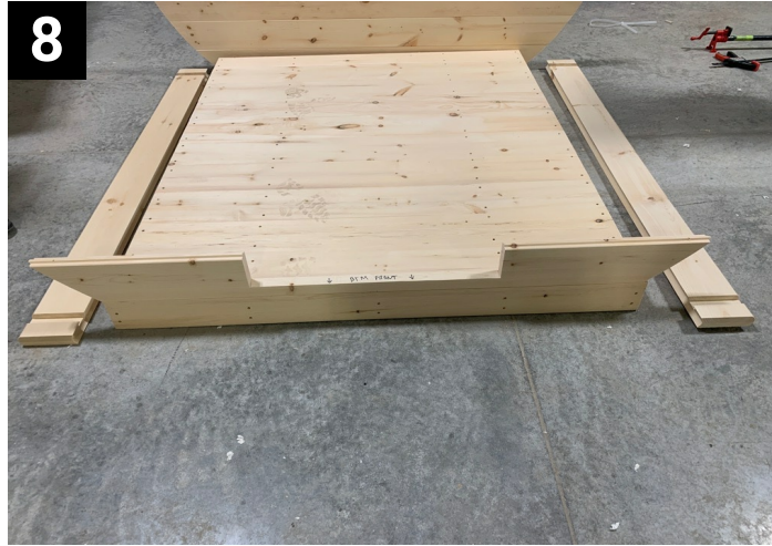
8 Lay front wall door pc on floor
