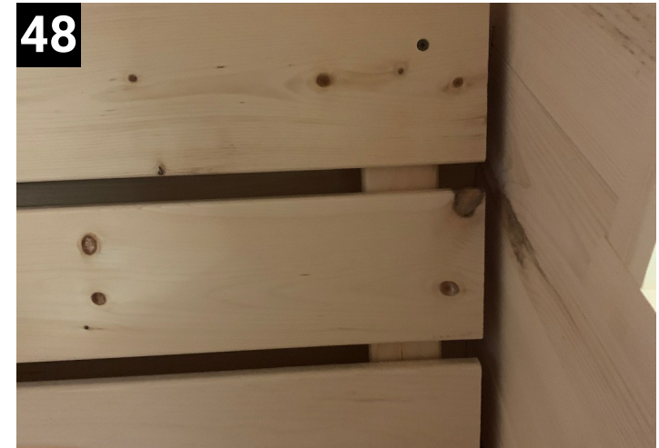
48 Fasten back rest with screw into pre drilled holes
