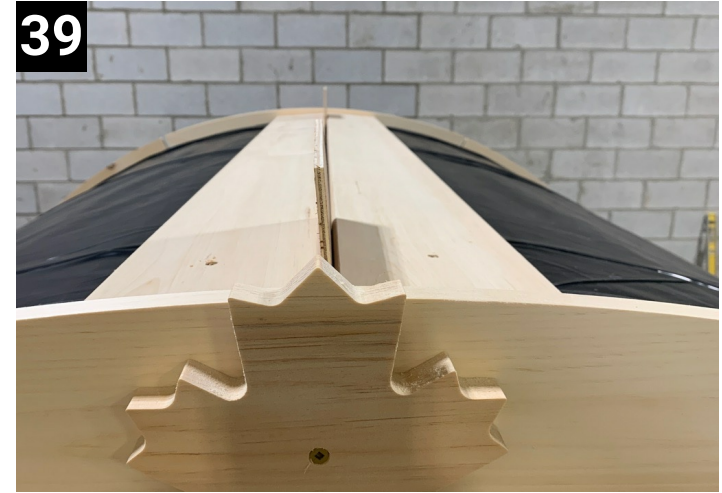
39 Vent is Center. Put 1/4" space between top 2 roof boards on Center.
