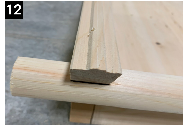
12 Put board tight to wall and fasten with 1 screw.
