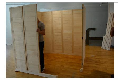
**STEP 11** - Install (1) of the narrow wall elements (N) on the other short wall (this will connect to the wall element you installed in step 3.)
