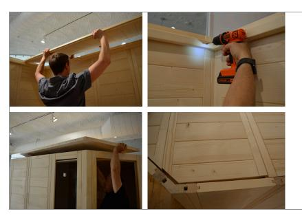
**STEP 18** - From the top of the sauna lay the (3) roof element sections in place. The side to face "up" is indicated, and the placement of the sections is intuitive. It is not necessary to screw the roof sections to the supports. A proper sauna needs airflow and should not be airtight. However, if your roof sections are not laying flat and if you can see gaps of light between the roof sections and the roof supports you can screw them down as desired to tighten the fit.
