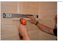
**STEP 19** - You will now install the bench supports. On the shorter left sauna wall and longer right sauna wall of the sauna, from the floor measure 34" and make a pencil mark. Position the top of the 23" upper bench support at the mark and use a level to insure that the support is level to the ground. Then screw the upper bench support into the wall element sections using 5x70 screws. Do this with both the right and left bench supports.
