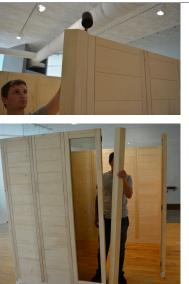
**STEP 13** - Install the (2) 45° corner posts to the narrow wall elements (one wood, the other glass) that frame the door opening. Once the corner post is in place you can nudge it into place with a rubber mallet.
