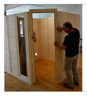
**STEP 16** - In the same way you installed the 45° corner posts, you will now install the doorframe. Raise both sides of the doorframe - you MUST use two people and keep the doorframe level – several inches above the 45° corner posts and then follow the same procedure as in step 13.
