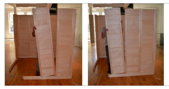
**STEP 10** - Continue to assemble the front short wall by adding (2) of the narrow wall element sections (N) followed by (1) of the narrow wall element sections with the edge clips facing to the door opening.
