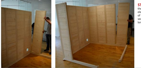
**STEP 8** - Continue the addition of wide wall elements (W) by adding (4) of the wide wall element sections along the second long rail.
