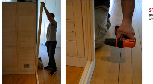
**STEP 7** - Place another 90° corner post to the end element and secure with 6x20 screws.
