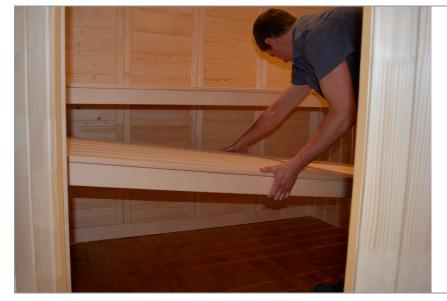
**STEP 23** - Place the lower bench on the lower bench supports. Since the lower bench is intended to slide in and out (it can be used as a step or as a full bench) it is not to be screwed into place.
