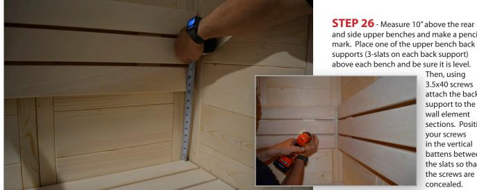
and side upper benches and make a pencil mark. Place one of the upper bench back supports (3-slats on each back support) above each bench and be sure it is level.
