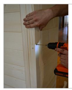
**STEP 5** - Using a cordless drill with the appropriately sized bit (included) use 6x20 screws and secure the 90° corner post to the short and wide element.
