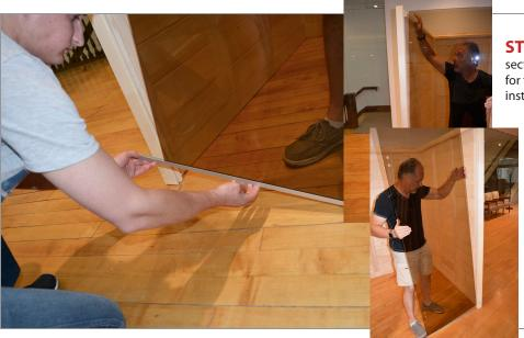
**STEP 15** - Locate the two glass window sections noting that one of them has holes for the door hinges. The instructions show installation with the door opening from left to
