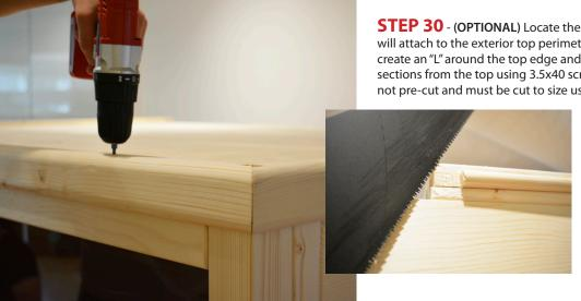
**STEP 30** - (OPTIONAL) Locate the exterior roof trim pieces. These will attach to the exterior top perimeter of the sauna. The pieces create an "L" around the top edge and will be screwed to the roof sections from the top using 3.5x40 screws. NOTE: The trim pieces are not pre-cut and must be cut to size using a hand saw. If the sauna is
