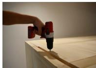
**STEP 18** - From the top of the sauna lay the (3) roof element sections in place. The side to face "up" is indicated, and the front roof section will fit into the groove of the header, and the rear roof section has a smooth edge. Once the roof sections are in place you can screw them to the roof support rails with 5x70 screws.
