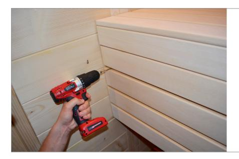
**STEP 26** - Position the lower back support (5-slats) against the vertical supports you installed in step 25. Holding the lower bench support tight to the top bench, attach to the vertical supports using 3.5x40 screws.
