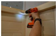
**STEP 13** - You will now install the roof support rails. Locate the (3) roof support rails and cut to length. The left and right rails should butt up to the front corner posts and the rear wall. NOTE: BE SURE THERE ARE NO GAPS BETWEEN THE WOOD WALL ELEMENTS BEFORE TAKING YOUR MEASUREMENTS.
