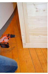
**STEP 9** - Add a wall section on the left wall and attach to the 90° corner post with 6x120 screws.
