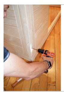
**STEP 4** - Verify that the element wall sections are square to the rails, perpendicular to each other, and that the flat top of the wall elements and corner posts align.
