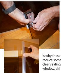
**STEP 31** - Install the hinges onto the glass door and secure to the window. The hinge consists of the hinge bracket, hole spacers, bracket cleat and hex screws. Be sure the screws are snug before mounting the door. NOTE: There is an intentional gap between the bottom of the door and the floor as well as between the glass panels. A sauna must have airflow, which
