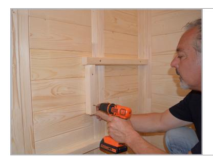
**STEP 25** - You will now install the lower bench back support. From the front of the two UPPER bench supports that you just installed, measure 1-1/2" back and make a mark. Then, install the two lower backrest supports (one on the left and right side of the sauna) to the sidewall element sections using 5x70 screws.
