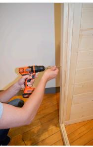
**STEP 8** - Add the third 90° corner post and secure with 6x20 screws as with the other rear corner post.
